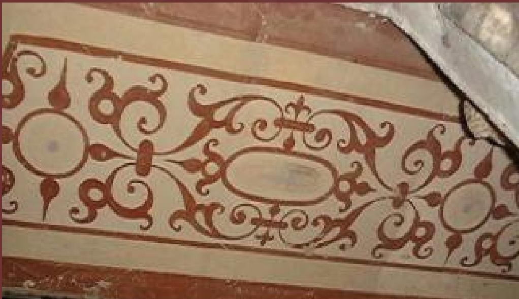
Upper lintel of window embrasure
